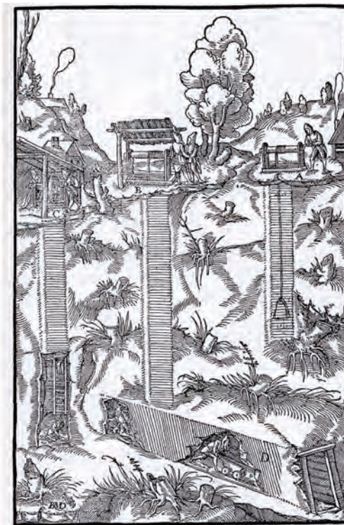
THREE VERTICAL SHAFTS, OF WHICH THE FIRST, A, DOES NOT REACH THE TUNNEL; THE
